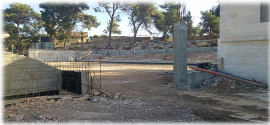
Work at Basketball Hall Just started
