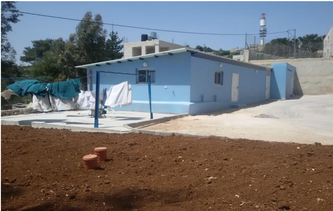
The newly constructed laundry section
